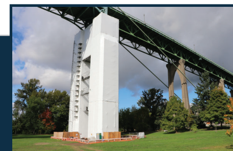
A column wrapped during construction under the St. Johns Bridge.
