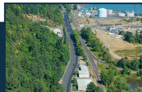
An aerial shot of U.S. 30 during construction.
